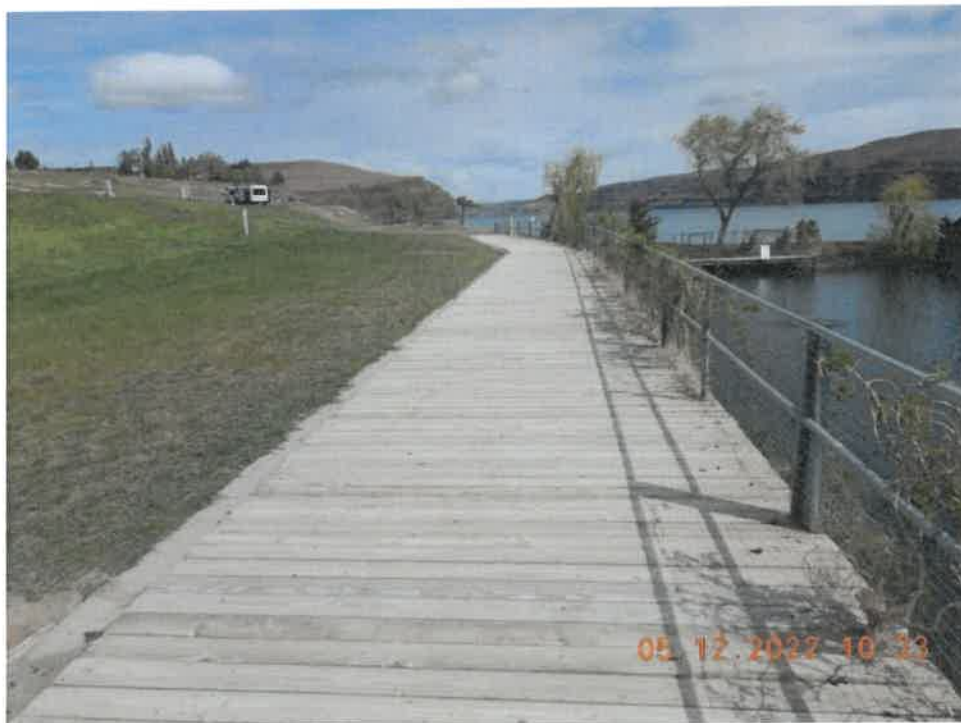
Photo 1: Overall View of Upper Boardwalk – Looking North
